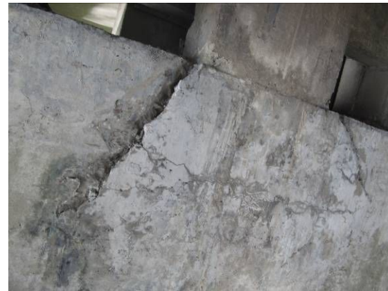
31#盖梁砼严重崩裂
